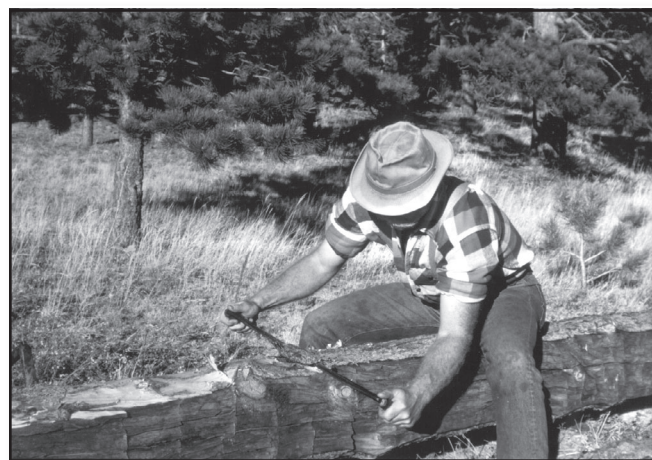
Figure 95—Removing bark from a green log with a drawknife.
